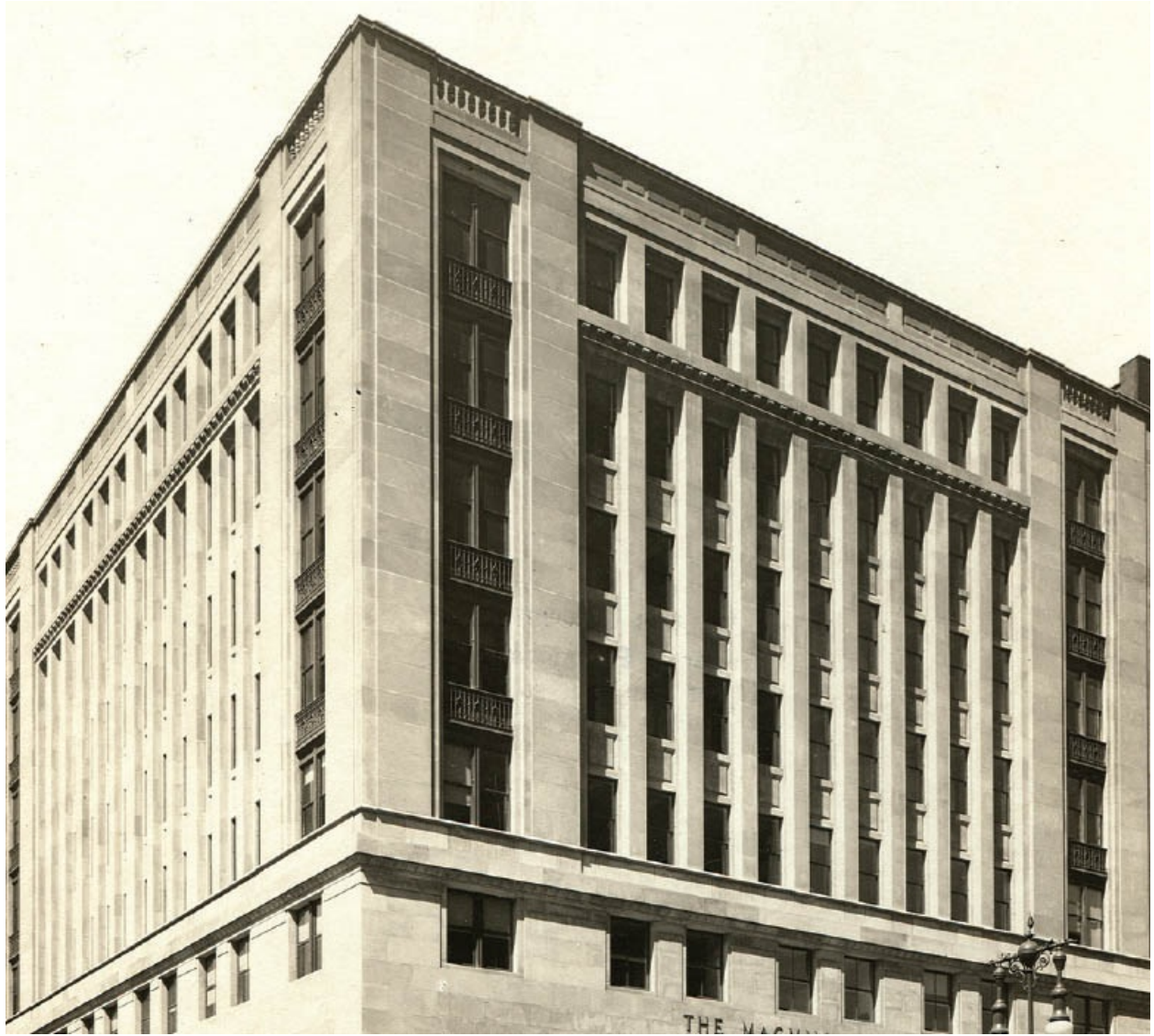
Macmillan Company Building , New York, 1924. This early skyscraper employs vertical elements that span the upper stories of the building. The horizontal elements sit back behind the vertical surface, establishing a second plane that appears to pass continuously behind the front plane, like the threads in a plaid fabric. Architects: Carrère and Hastings with Shreve and Lamb. Vintage photograph.
