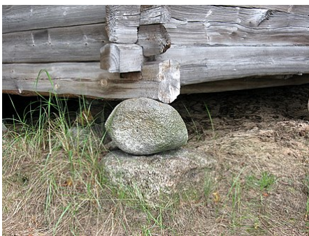
The simplest foundation, a padstone. The Ethnographic Open-Air Museum of Latvia
